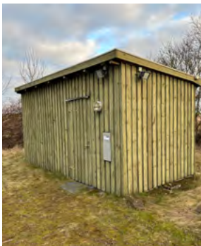
Den gamle pumpestation
